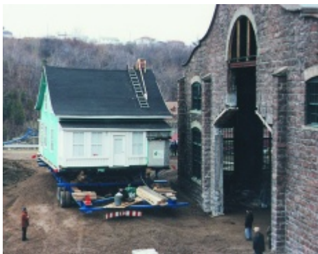
Villeneuve's home being moved in November 1994.
